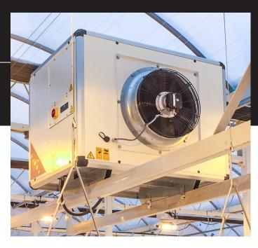
A dehumidification system is a more **cost-effective way to control humidity** than venting outside air, as the highest humidity points inside the greenhouse often correspond with the lowest outside temperatures, leading to higher heating costs to maintain greenhouse temperature.
