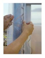
This clip system has been tested and will withstand loads of upto 260kg/m2, which exceeds New Zealands Very High Wind Zone rating of 180km/hr wind speed, or 158 kg/m2 of wind pressure. This has been formulated using NZ4211.1985 using Ultimate Wind Pressure (UWP).
